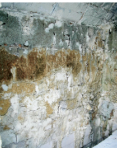
Kiln #2 after 80 firings. Sides and back walls.
